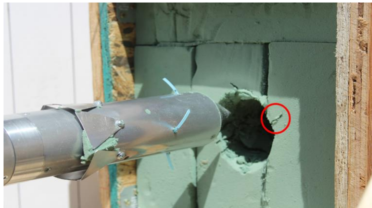
Figure 3.6: Root System Pullout Test
